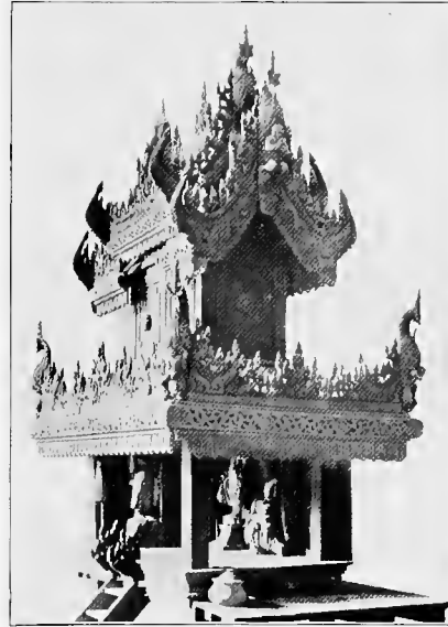
63. DETAIL OF EAVES AND GABLE.
